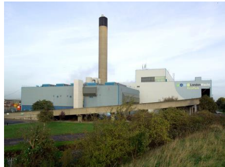
Energy from waste facility
